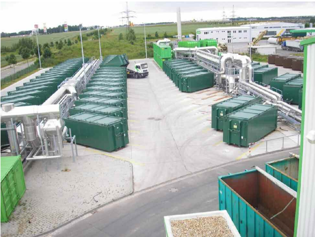
Figure 3 Stabilisation in composting containers, thermal exhaust gas cleaning and biofilter
