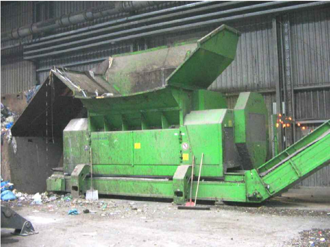
Figure 4 New pre-shredder in Stralsund
